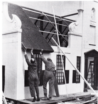
■ Fitting a section of Fibre-Thatch roofing to the Union-Castle/Satour display stand during final stages of construction. The glass-reinforced fibre thatch gives a visual effect similar to straw and reed, and is easy to handle.
